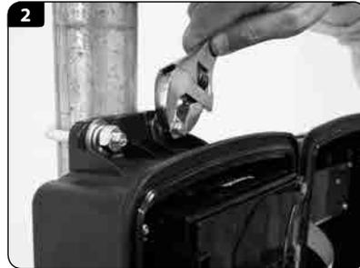
3. Carefully attach an electrical conduit adaptor (*Clipsal 50mm or Carlon 1 1/2"*) to the XCI device.
