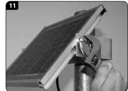
11. Now tighten the M8 nuts on each side of the mounting bracket to secure.
